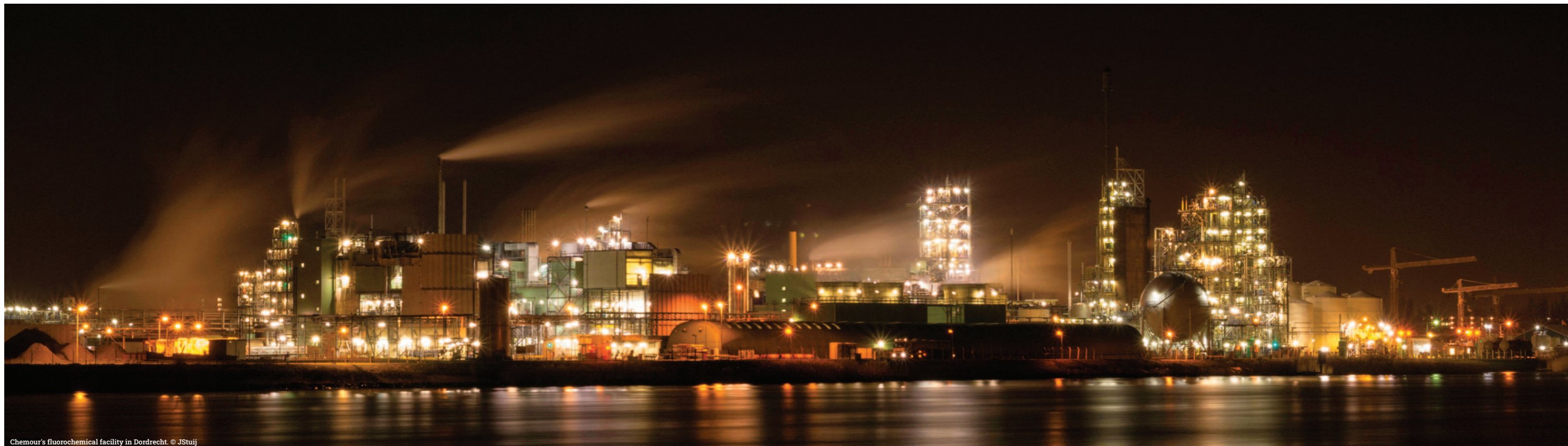
Chemour's fluorochemical facility in Dordrecht. © JStuij
