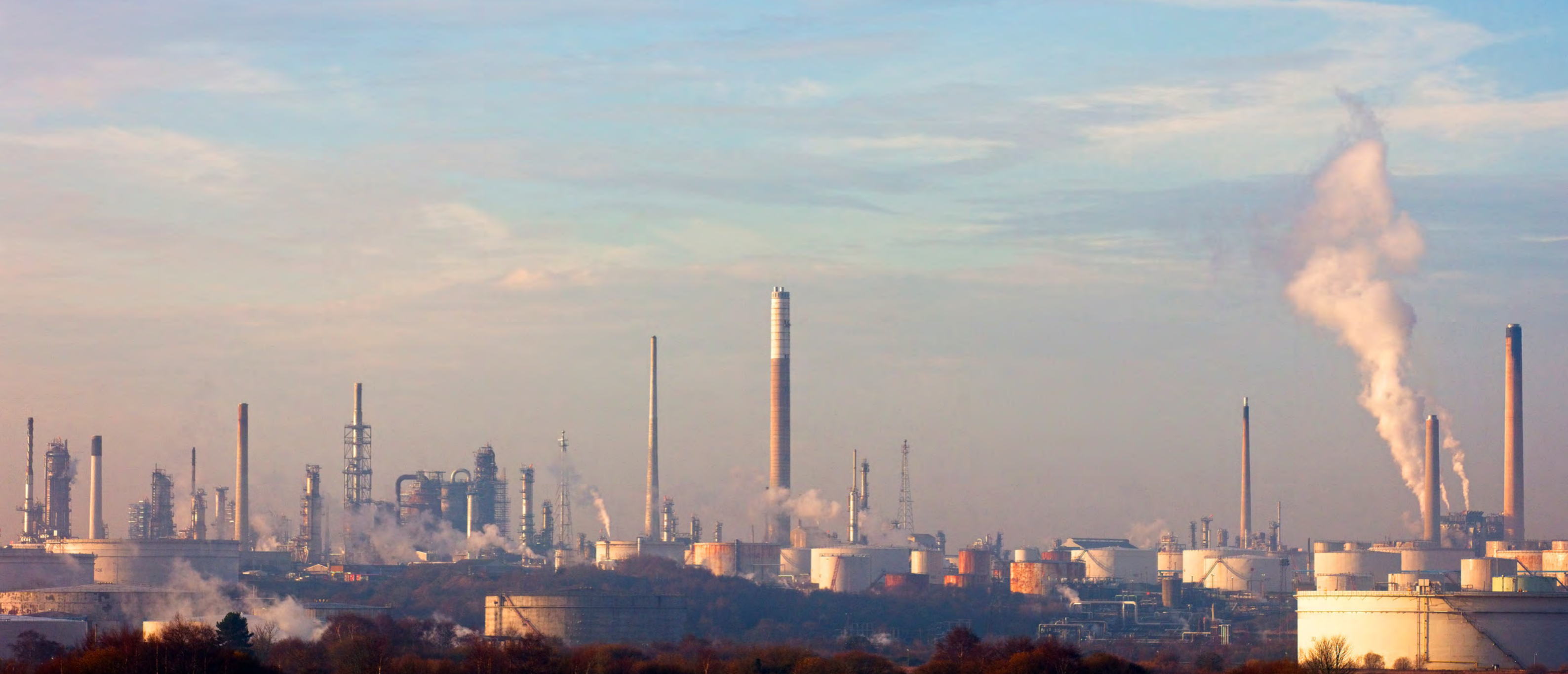
Above: Oil refinery and petrochemical complex
